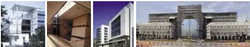
2 • 1 - Euralille Towers Lille, France • 2 / 3 - French Embassy Singapore • 4 - Caisse d'Epargne National Headquarters, Paris France • 5 - The Putrajaya, Urban Design and Civic Centre Complex, Malaysia; Photos: Nicolas Borel
